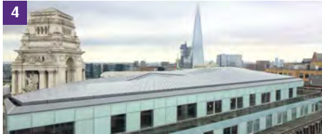
4 Trinity Square – Offices
